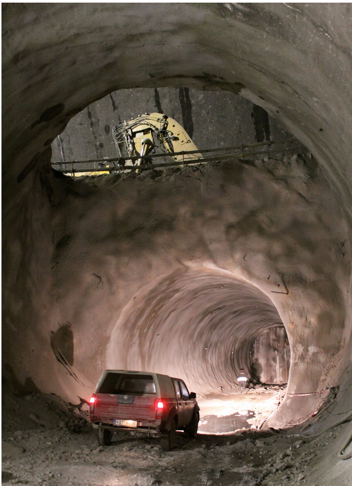
Fig. 9 – The Blanka Tunnel – the Crossing of the Tunnels Excavation
