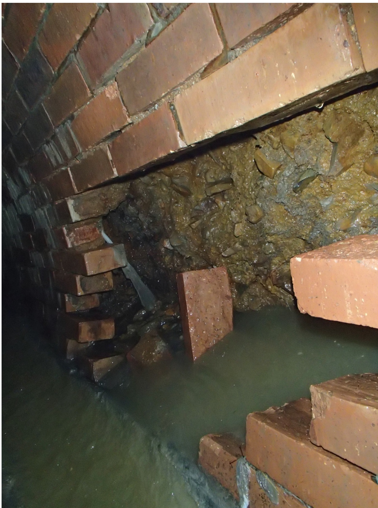
Fig. 8 – A cavern detail, length between the Š6 and Š7 shafts (photo by INSET)
