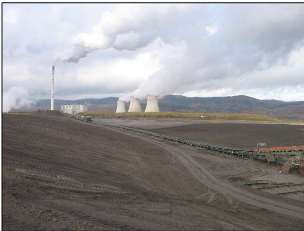
Figure 3. Earth structure which was compacted by a roller without vibration.
