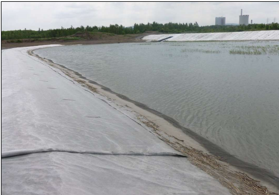
Fig. 7. New earth dike and flooded cassette – a coal power plant in the background.
