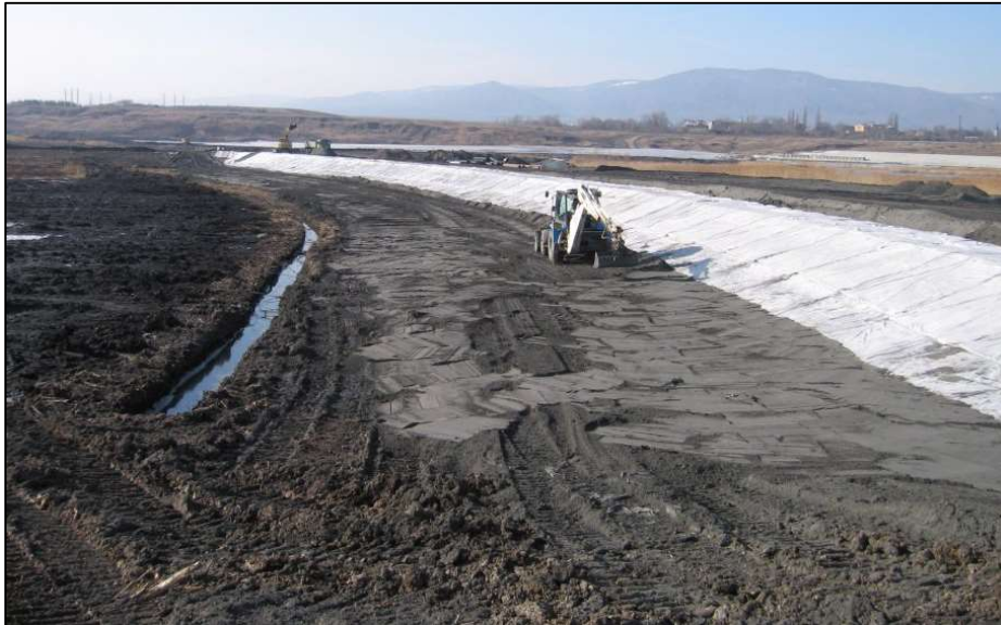
Fig. 6. Construction of a new earth dike.
