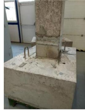
Step 4-Applied repair mortar
