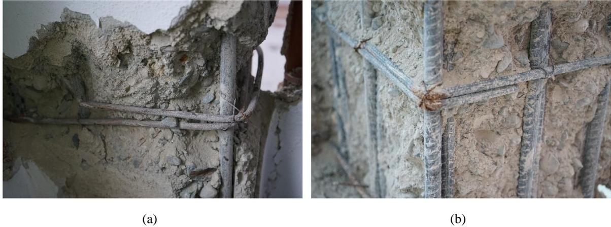
Fig. 1.8. Hook details of seismic hoops in column (a) plain round bars (b) deformed bars (Yurdakul et al. 2021).
