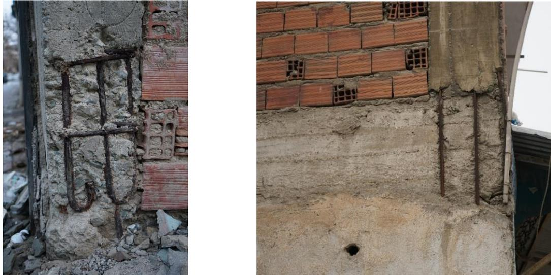
Fig. 1.12. Corroded reinforcement (Yurdakul et al. 2021).
