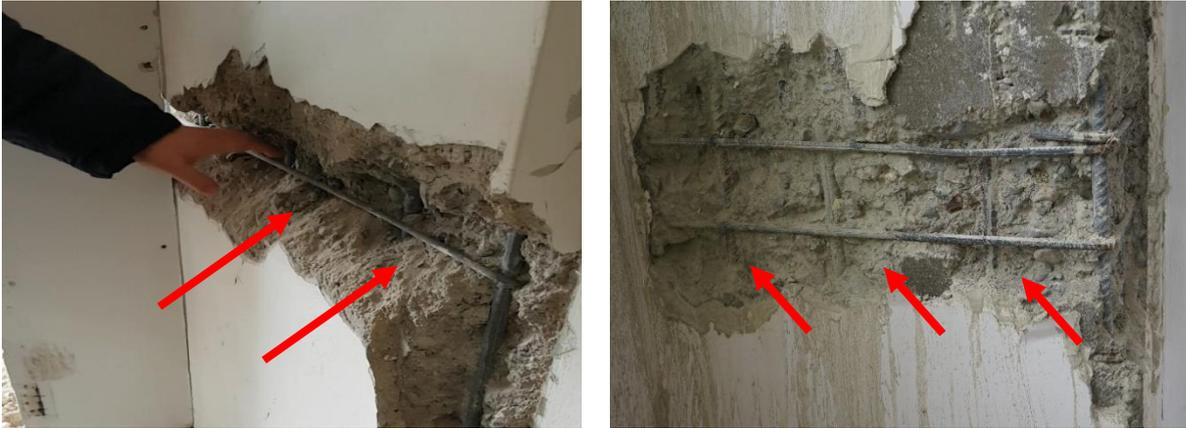
Fig. 1.10. Reinforcing detail without cross-ties (Yurdakul et al. 2021).
