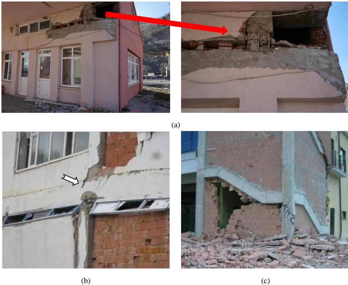
Fig. 1.19. Short column due to structural element (a) Elazığ 2020 earthquake, Turkey (Yurdakul et al. 2021) (b) Van 2011 earthquake, Turkey (Öztürk 2015) (c) L'Aquila 2009 earthquake, Italy (Ricci et al. 2011).
