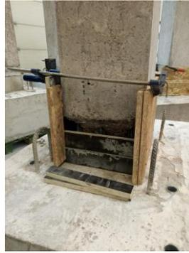
Step 3-Formwork for repair mortar
