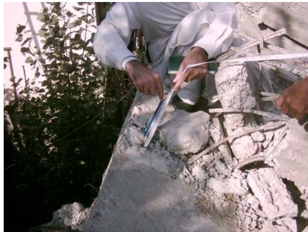
Fig. 1.11. Reported lap splice failure by Naseer *et al.* (2010).
