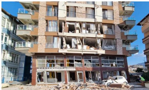
Fig. 1.13. Soft story induced damage in Maraş Earthquake 2023 (Photo Credit: Yunus Demirtaş)
