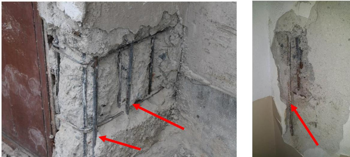
Fig. 1.9. Unengaged longitudinal bar (Yurdakul et al. 2021).
