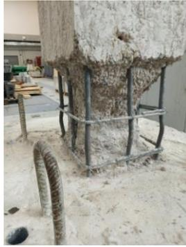
Step 2-Removing the loose concrete
