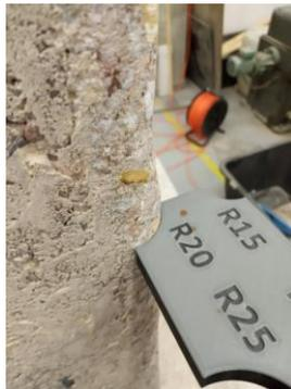
Step 6-Rounding sharp corners on column
