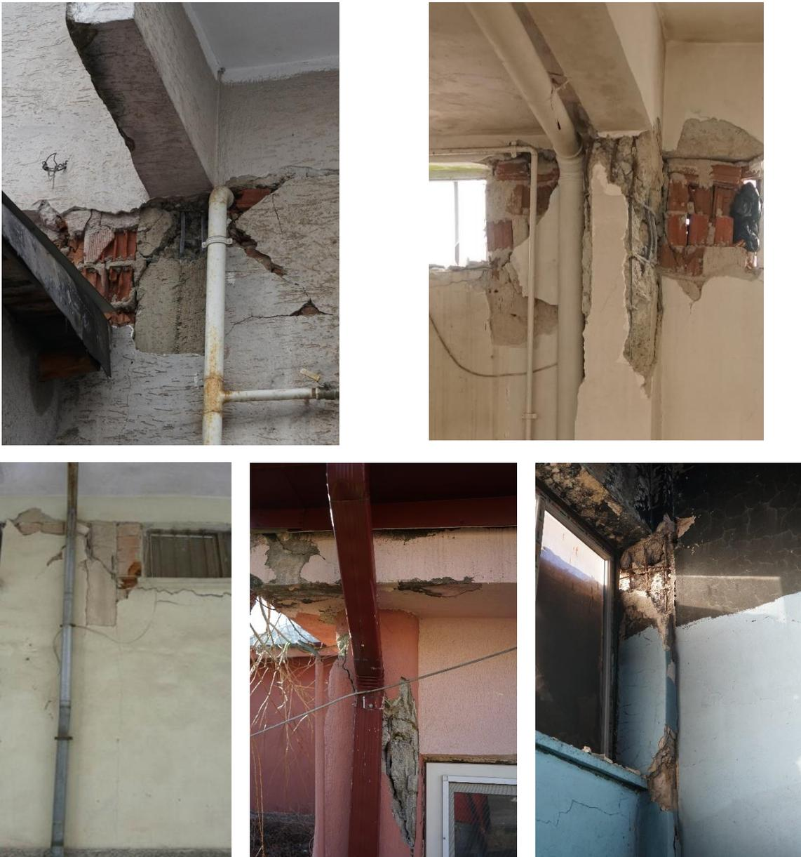
Fig. 1.20. Captive column due to ribbon window (Yurdakul et al. 2021).
