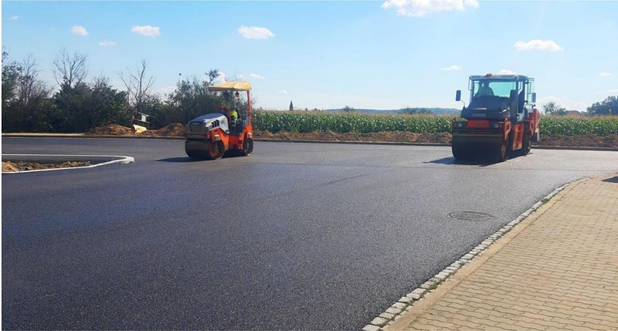
Figure 8. Paving the rest station Rajhrad at D52 motorway with ResiSkan in 2020.
